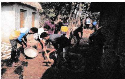
(Soak Pit Construction)
