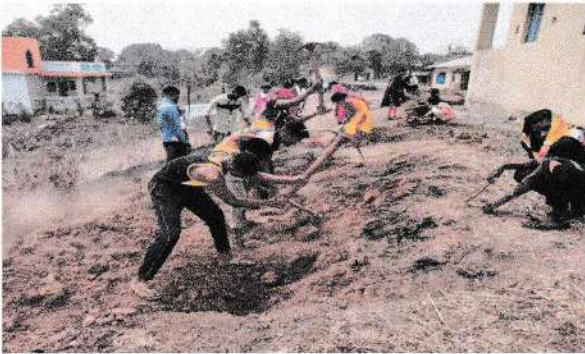
(Soak Pit Construction)
