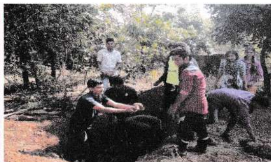
(Soak Pit Construction)
