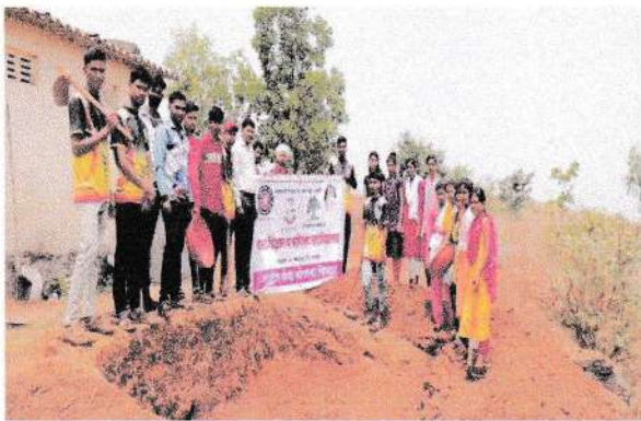
(Compost Pit Construction)
