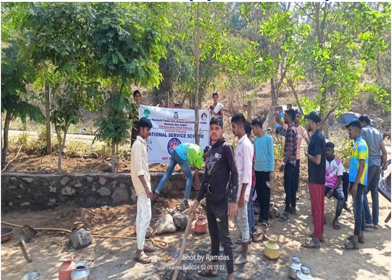
NSS Students completed a wall compound to Z P School
