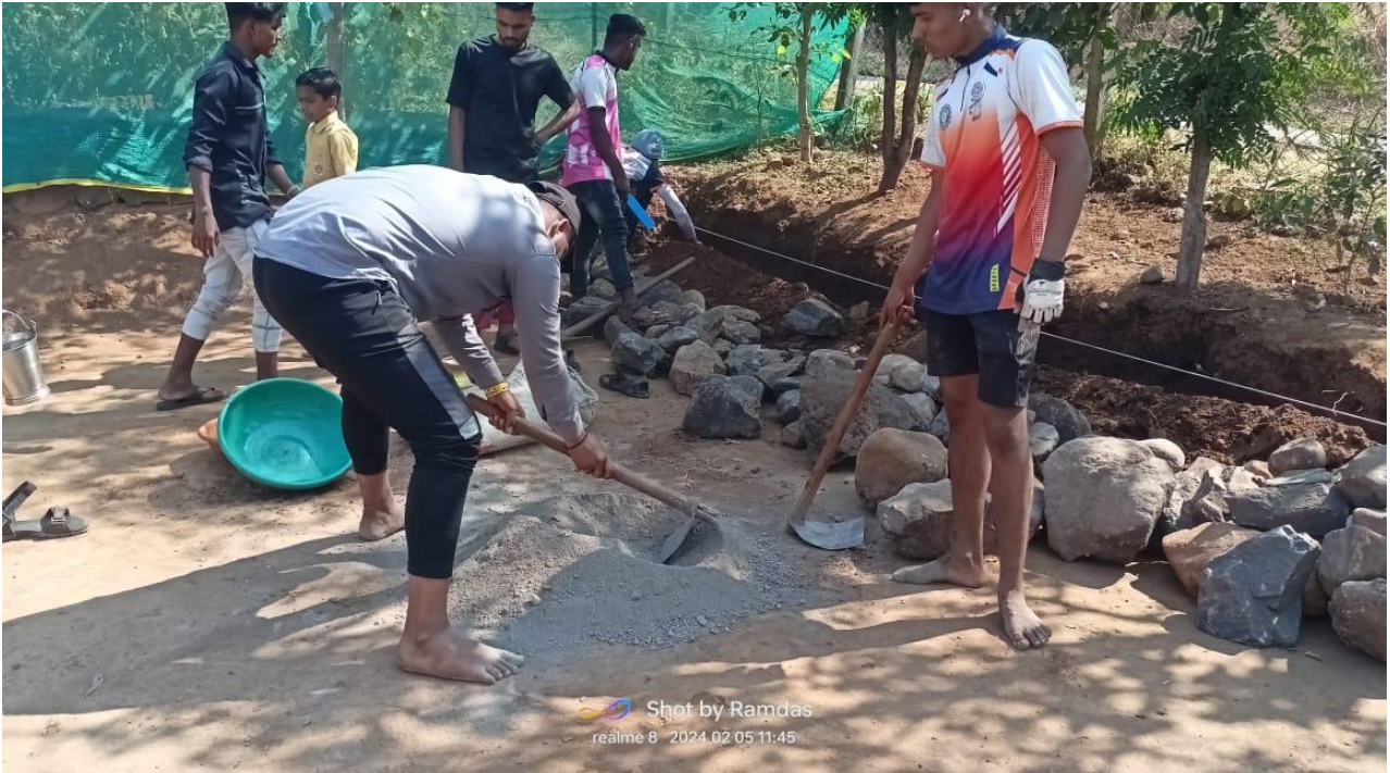
Participated students in wall compounds preparation at school
